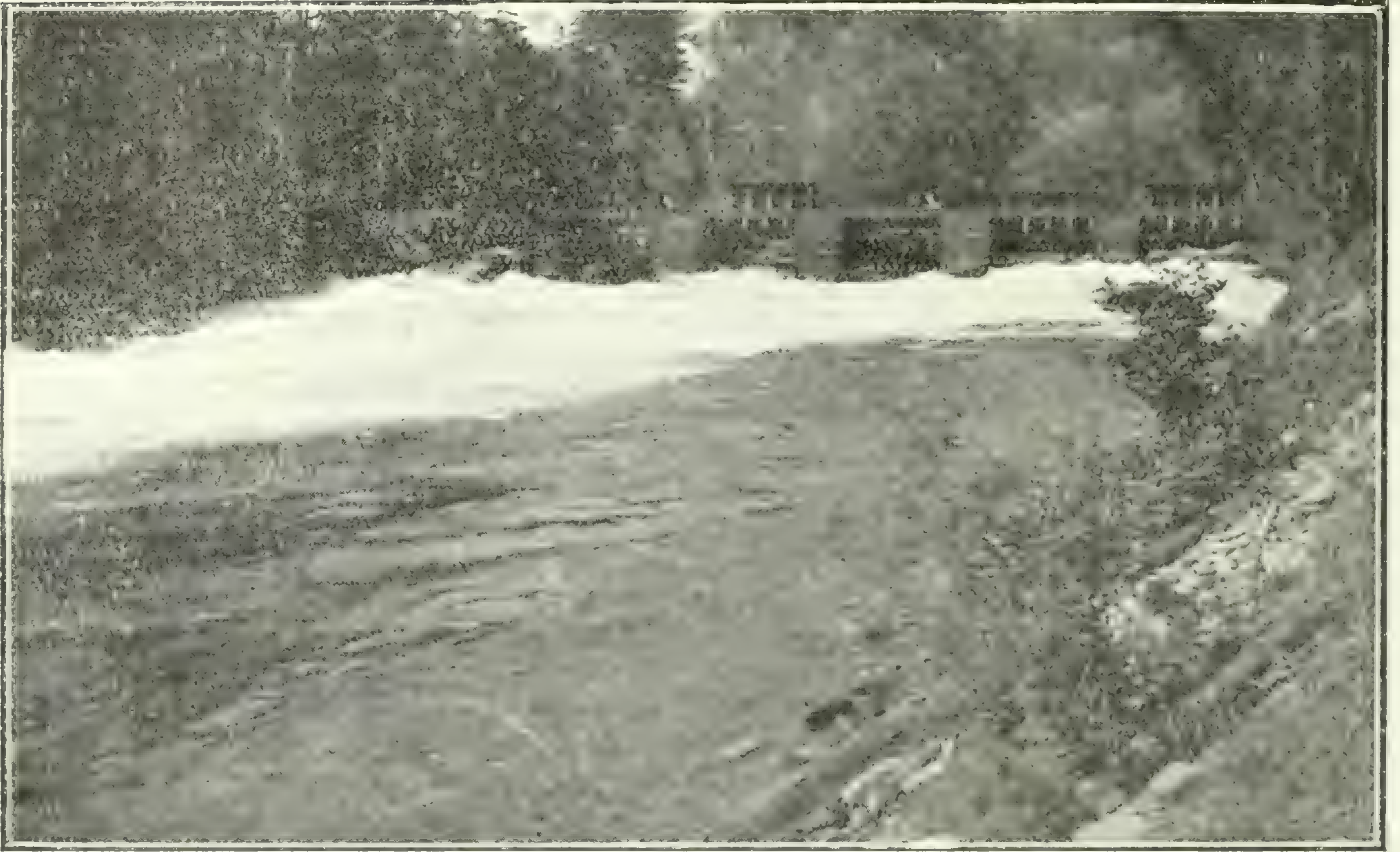
Adams River—Adams River Lumber Company's Dam below Adams Lake.
